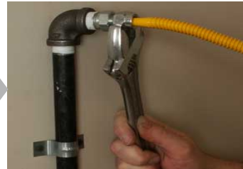
Stage 3 – Modification of Heating System
