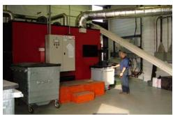
total demand of County Hall. Over the 2005/6 heating season, the boiler has so far supplied 1,138,140 kWh of heat generated from over 400 tonnes of wood chip, equivalent to a reduction of the emission of 216 tonnes of CO<sub>2</sub>. In total, some 700 tonnes of carbon dioxide emissions have been avoided over the first four years of operation of the wood burning system.
