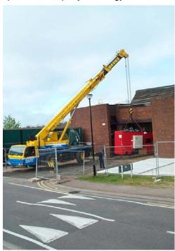
company supplied, installed, owns and operates the boiler plant, which produces around 1.3 million kWh/year of heat from between 500 and 600 tonnes of biomass fuel. Heat is measured by a certificated
