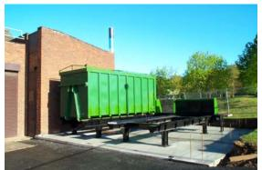
system, with two 35m<sup>3</sup> steel containers for storage. Each container holds about 9 tonnes of fuel, and the plant burns up to 20 tonnes per week at full load. There is no tipping on-site and no underground bunker, merely a flat concrete pad.
