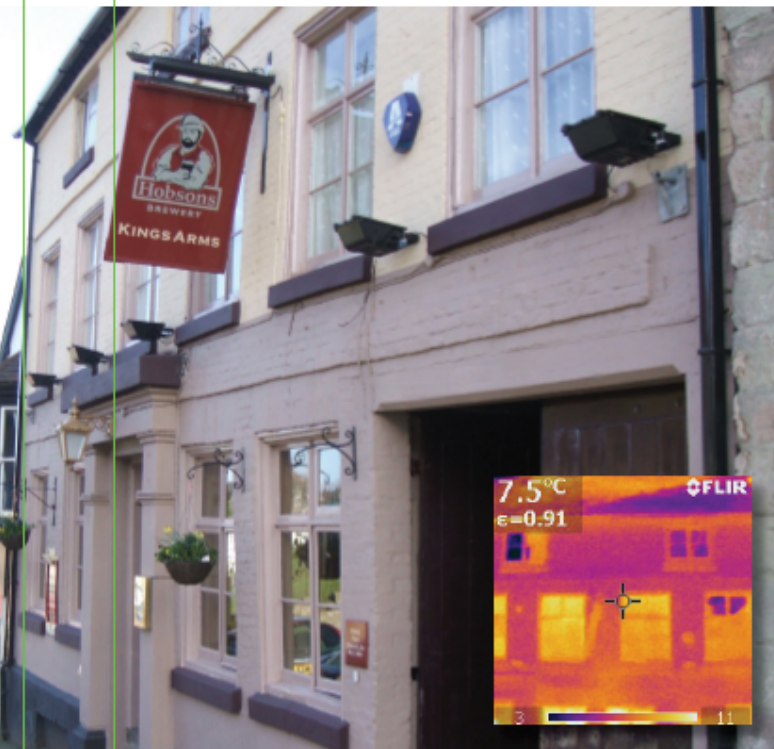
The thermal image above shows bright yellow-orange patches where heat is escaping from the hotel.
