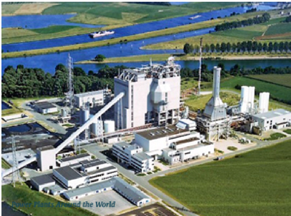
Buggenum IGCC, Holland (Pre-combustion capture * does not include CCS)
