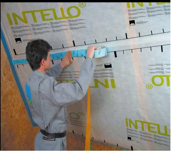
Connections of corners and edges in timber construction
