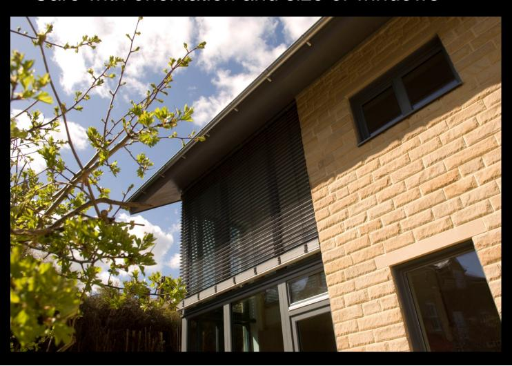
Superinsulation – wall, floor and roof U values c. 0.1W/m2K
