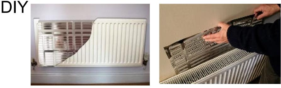
The rad reflector panels have an undulating surface that cause a disturbance to the convected airflow, which cause it to turbulate and fall to a lower level sooner, making the room more evenly temperate
